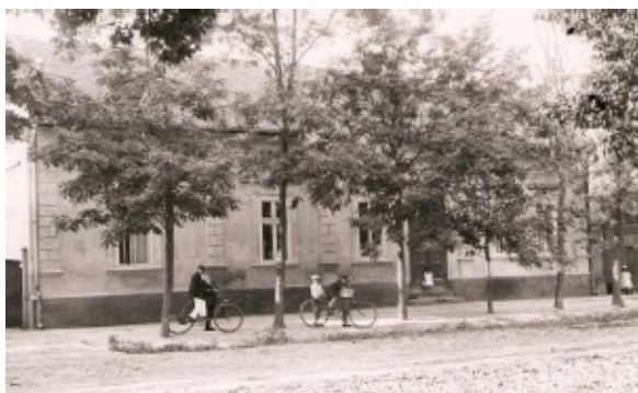
Figure 2 Kuzura Klein House (front)
